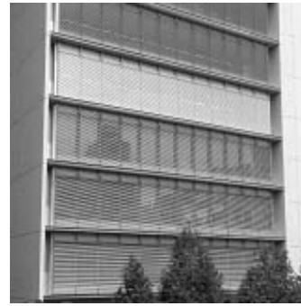
Fig.13: West façade of building
