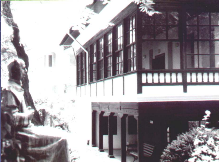
South façade and inside porch, built in the Theodor Pallady Museum, Campulung Muscel
