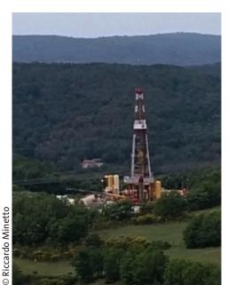
View of the Venelle-2 well. The well was designed to sample supercritical fluids.
