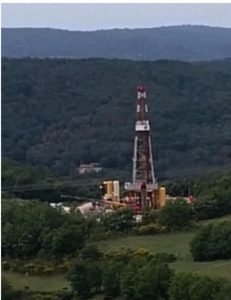
View of the Venelle-2 well. The well was designed to sample supercritical fluids.
