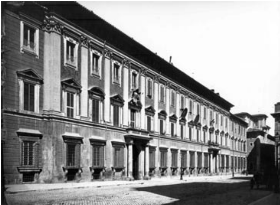
Fig. 4. Facade of Palazzo Chigi-Odescalchi, Rome. (ICCD.)
