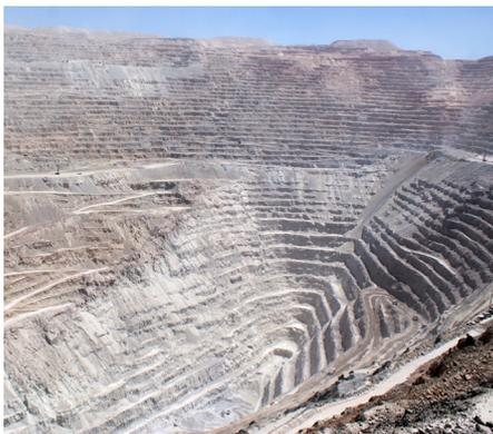
The Chuquibambilla open pit mine (Chile) exploits one of the largest porphyry copper deposits in the world: it is 4.3 km long, 3 km wide and up to 0.9 km depth.
