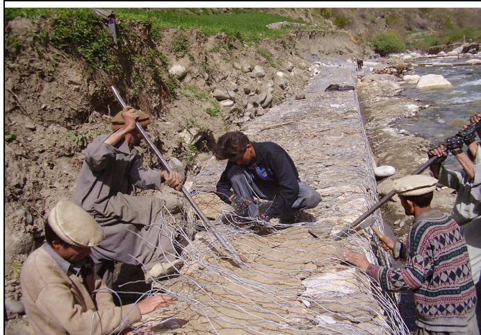
Fig: 20 Protective work along the river bank to protect the lateral erosion and bank collapse
