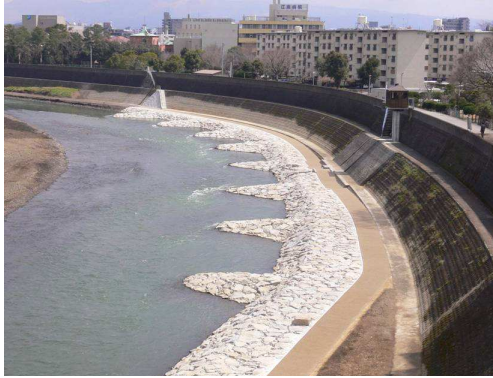
Figure 41 : Oe Area-Gravel Supported Dykes ( Personal Communication from River and Road Network office of Kumamoto City,2006)
