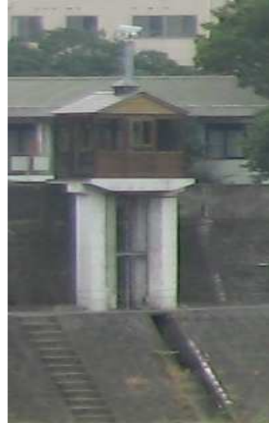
Figure 45 : Shirakawa river electronic announcement board and camera surveillance located on dyke ( Archive of Volkan ORAL on 20 October 2006)
