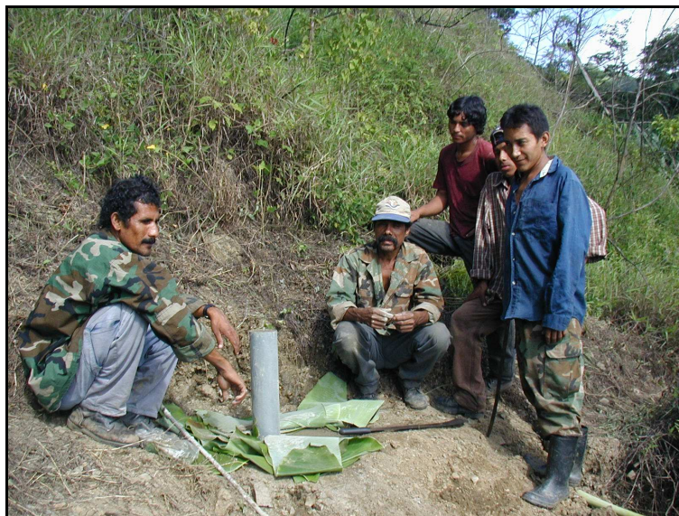
Photo 31: End of the construction; it will dry for the night under banana leaves.
