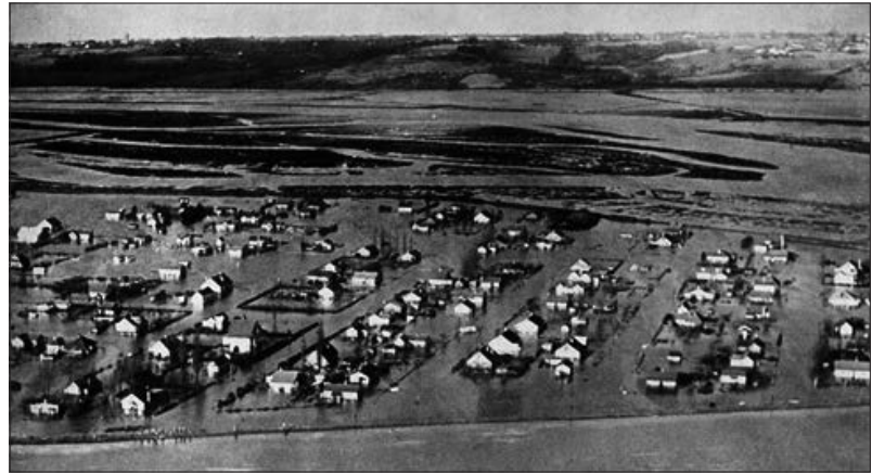
Figure 4: The extent of devastation, Canvey Island, Essex, 2 February 1953. Source: Grieve, H. 1959: The Great Tide: The Story of the 1953 Flood Disaster in Essex . (Essex: Essex County Council Press) p.292.
